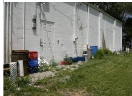
Figure 23: Material at Rear of Commercial Site
