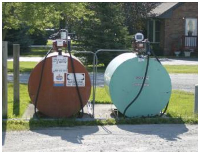
Figure 28: Lack of Containment on a Connected Impervious Surface
