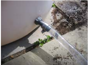
Lower hose barb and attached vinyl hose.
