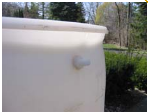
Upper hose barb for water overflow.
