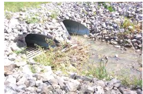
Longstaff Drain at Hayes Road
