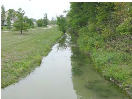
Harrington Drain at 14 Mile Rd
