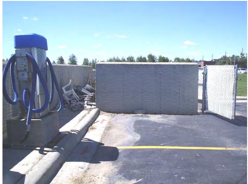
Dumpster Area on Impervious Surface with Debris on the Ground – Gas Station in Macomb Township
